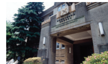
29 予防医学校舎 Building for Preventive Medicine & Public Health
