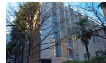
23 3号館(北棟) Building 3(North Wing)
