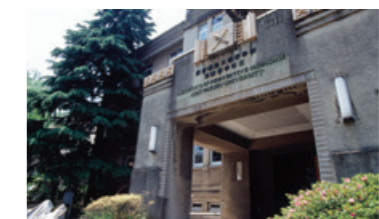
⑲ 予防医学校舎 Building for Preventive Medicine & Public Health
