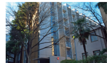
⑬ 3号館(北棟) Building 3(North Wing)
